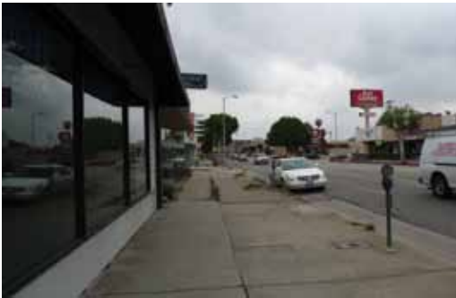
A sidewalk on Camden Avenue and Pico are full of cracks and weeds. (existing conditions shown above)
